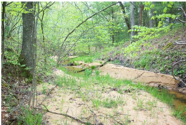
Overtopping of a small earthen dam during spring melt and heavy rains contributed tons of sediment to the East Branch of Tank Creek and eventually the Pere Marquette River.
